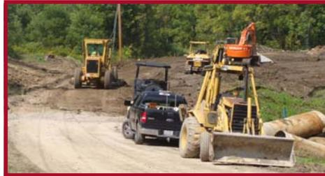
Carter's Corner Road is closed and work is underway to replace the Little Walnut Creek Bridge. The closure is expected to last until November 27. The project includes replacement with a new 36-foot span concrete slab bridge. Approximately 800 feet of the roadway approaches will be realigned to correct a sharp curve at the bridge.
